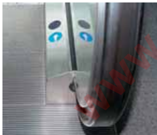
Traffic lights on decking
