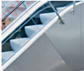
Stainless steel cladding
